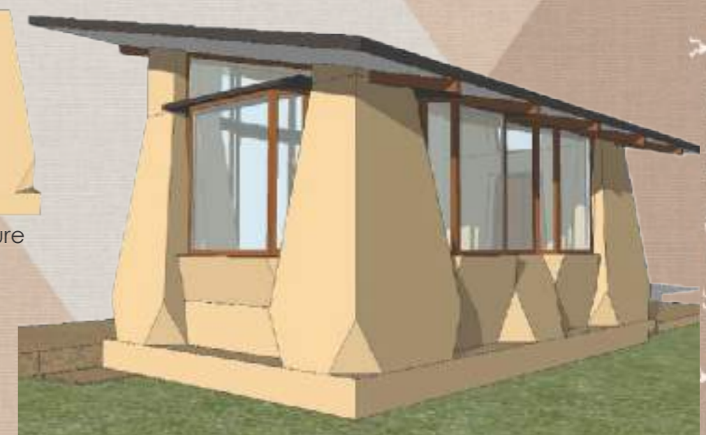
Completed Studio space covered using bamboo and sheet roof
